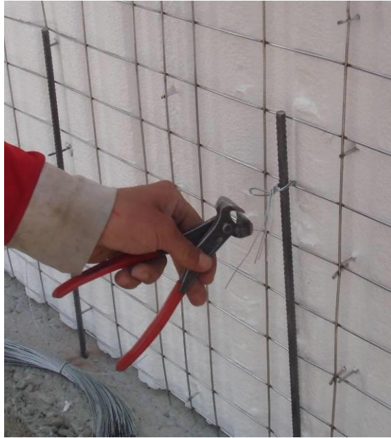
Figure A3.2. Tying panels with corrugated steel installation/foundation by means of wire. Example.
